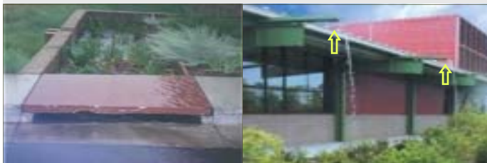
Stormdrain leading to bioretention cell
