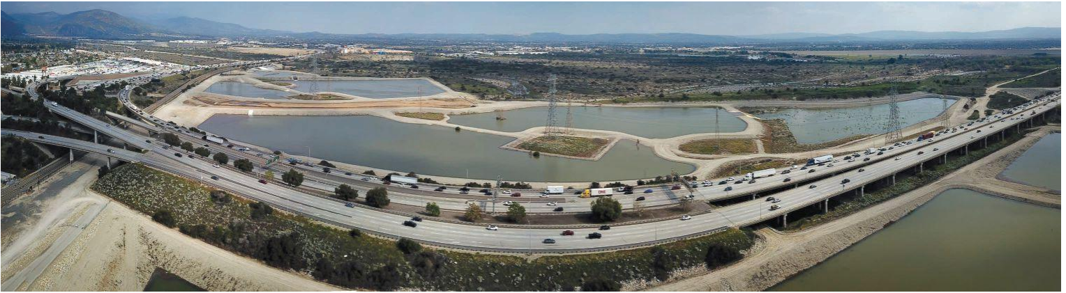
At left, an aerial view looking south shows the California Aqueduct (right) and the Delta-Mendota Canal (left) south of San Luis Reservoir near Los Banos in Merced County. The facility is part of the San Luis Joint-Use Complex, which serves the State Water Project and the federal Central Valley Project. Above, the Santa Fe Spreading Grounds, which are visible from the 210 and 605 freeways, is where water percolates into the Main San Gabriel Basin. Most of Upper District's water supply is from this groundwater basin with some imported via the State Water Project.
